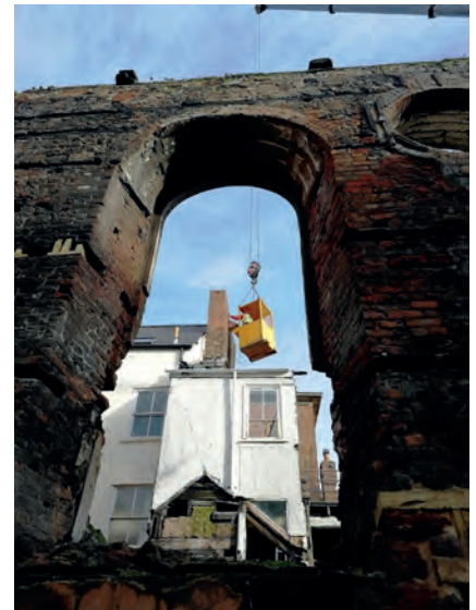
▲ Paul Williams preparing to fix the Trimble S9 to the wall
